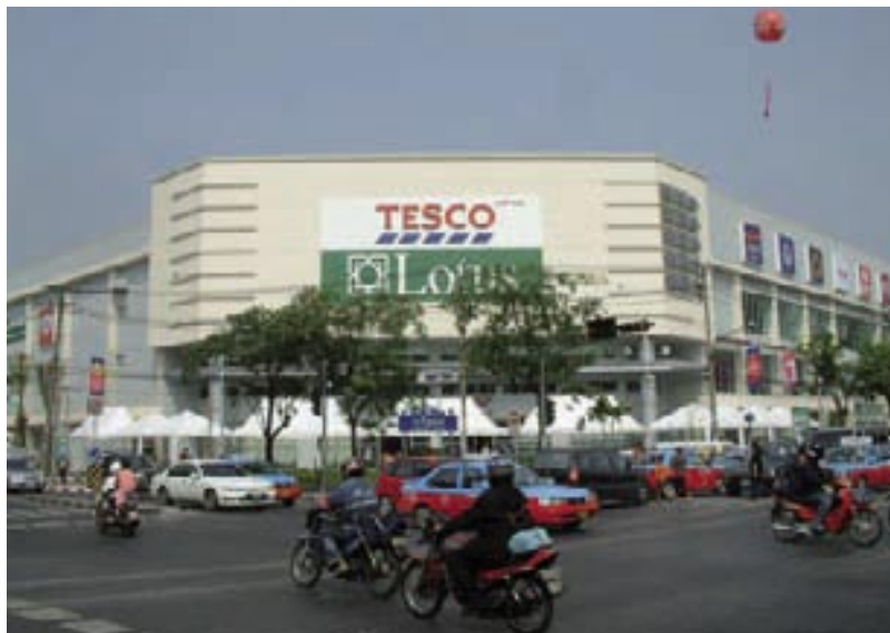
Tesco's growing network of stores in Thailand requires a powerful EMS to keep energy management under control
