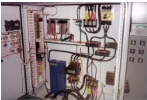
One of several Pump-PAK™ cabinets housing motor controls and PLC components.
